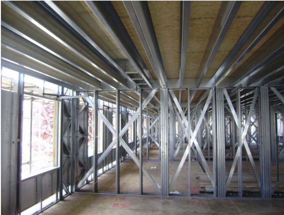
Figure 4.2 Light steel cross-walls and floor joists
