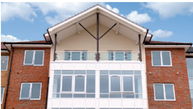
Figure 17 Ground supported balcony in a light steel care home building (Image courtesy of Kingspan Profiles and Sections)
