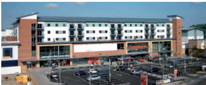
Figure 4 Light steel frame supported on a composite steel structure above a supermarket in Farnborough (Image courtesy of Metek UK)
