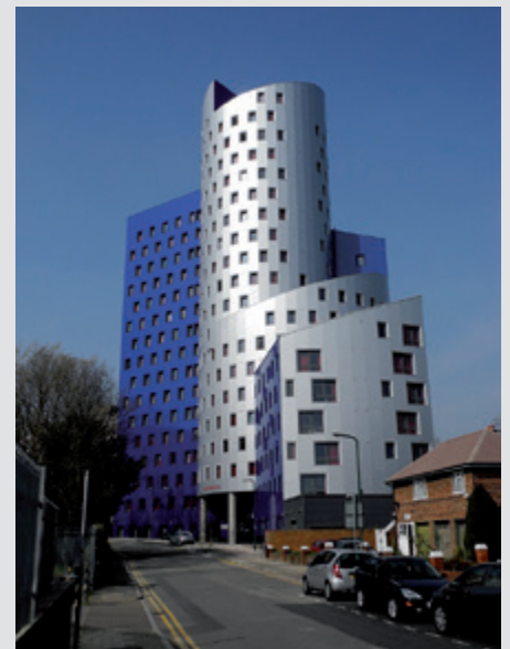
High rise modular residential building (Image courtesy of Ayrshire Framing and Futureform)
