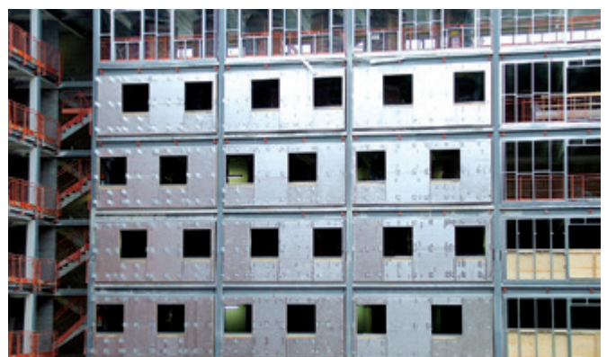
Figure 7 Prefabricated light steel infill wall panels used in a multi-storey steel-framed residential building (Image courtesy of Kingspan Profiles & Sections)
