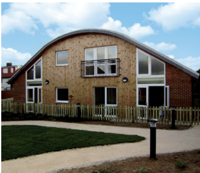
Figure 12 Code level 5 modular apartments in west London (Image courtesy of Futureform and Ayrshire Framing)
