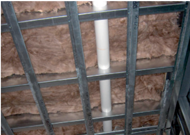
Figure 16 Services installed through openings in light steel floor joists
