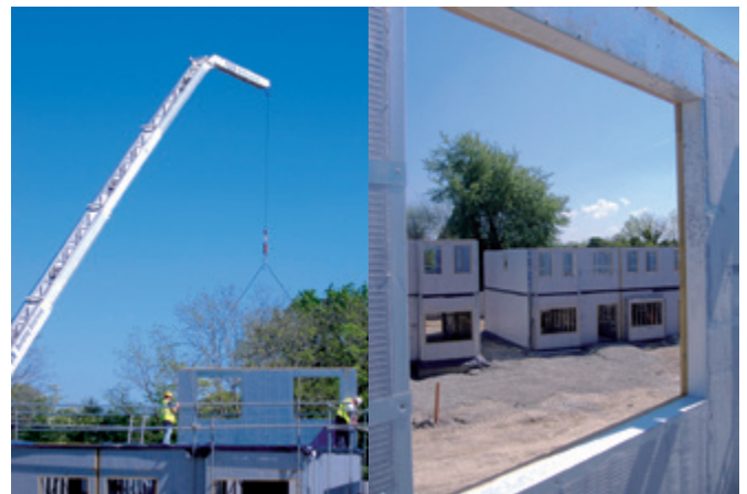
Figure 3 Pre-fabricated light steel wall panels with bonded insulation (Image courtesy of Fusion Building Systems)
