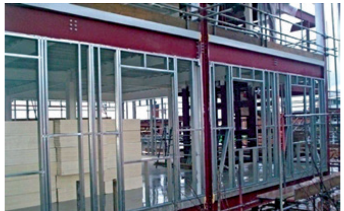
Figure 6 Light steel infill wall used in a multi-storey steel-framed residential building (Image courtesy of Metek UK)
