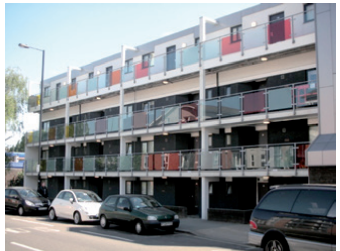
Figure 13 Building extension using modular units in London
