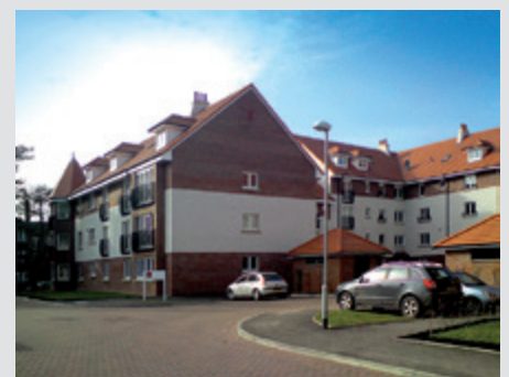
Light steel 4-storey residential building in Glasgow (Image courtesy of Kingspan Profiles & Sections)
