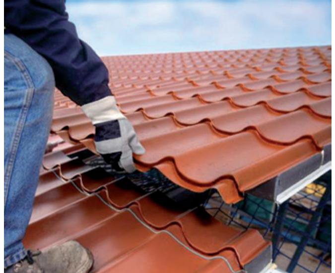
Figure 9 Composite panel with tiled finish supported on Z section purlins (Image courtesy of Kingspan Panels)
